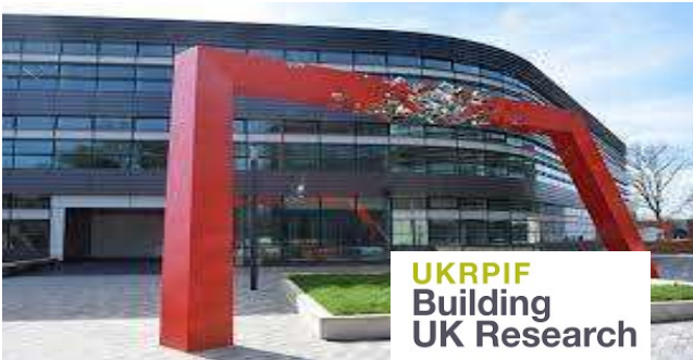
Li Ka Shing Centre, 2017
